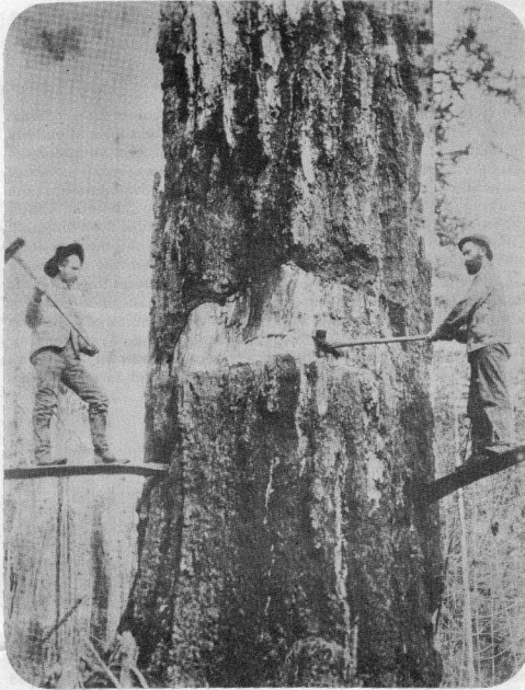
This historic picture shows a tree six feet in diameter and two hundred feet tall being felled to clear the site on which Vancouver, B.C. now stands. The "Bowling Pin" method was used in this operation. Smaller trees were cut half way through and then the giant tree was felled upon them. Two to three acres of forest went down in this way to one great resounding crash.
